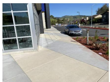
CONCRETE PAVING, BROOM FINISH, NATURAL COLOR, TYP. CONCRETE PAVING, BROOM FINISH, INTEGRAL COLOR, TYP.
